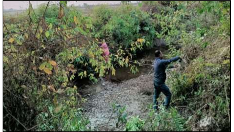
Water Harvesting Structure at Deolguri MWS-1
