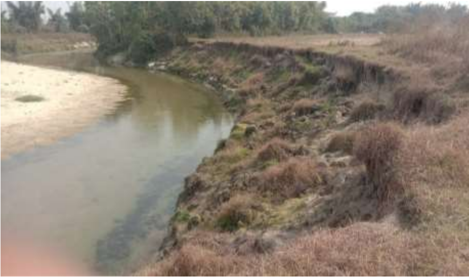
Boulder Pitching at Dangsibari village MWS-4
