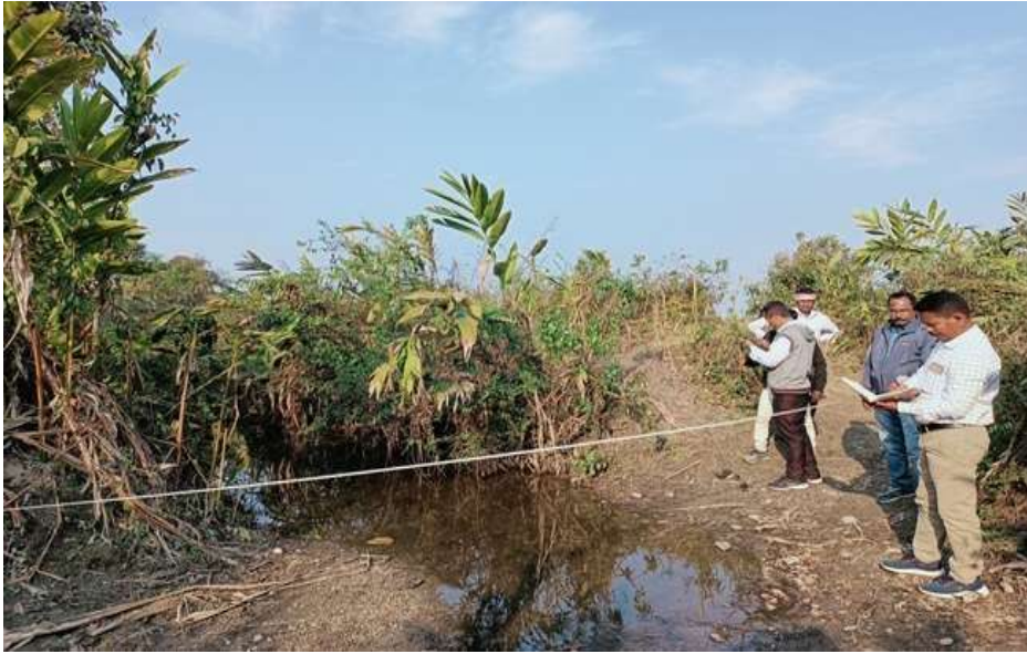
Gully Control Project at Balapara MWS-2
