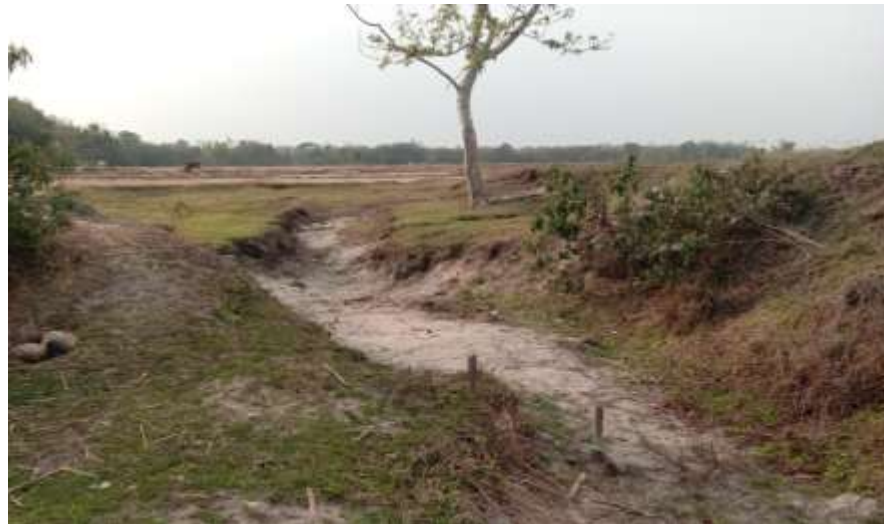
Gully Control Project at Bairajhora village MWS-4
