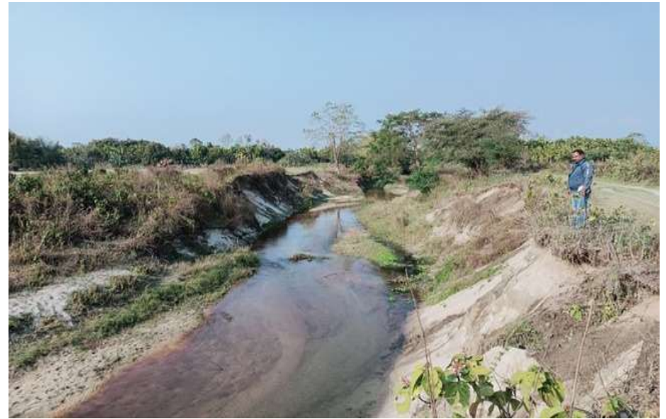
Boulder Pitching Project at Laoripara MWS-2
