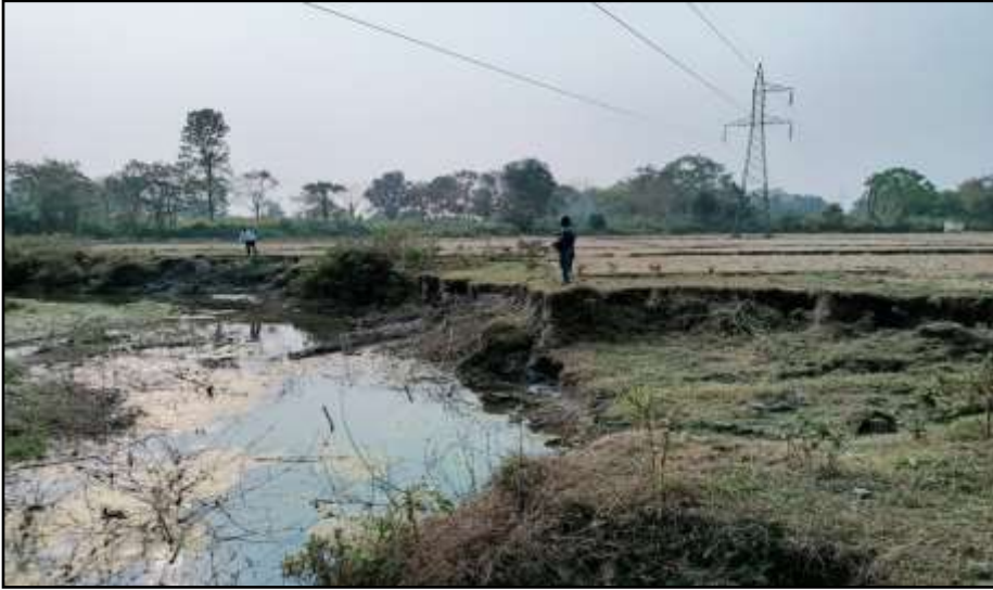
Boulder Revetment Work at Dologaoon MWS-1
