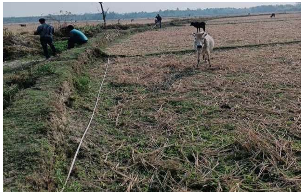
Const. Brick Channel at Solmari MWS-5
