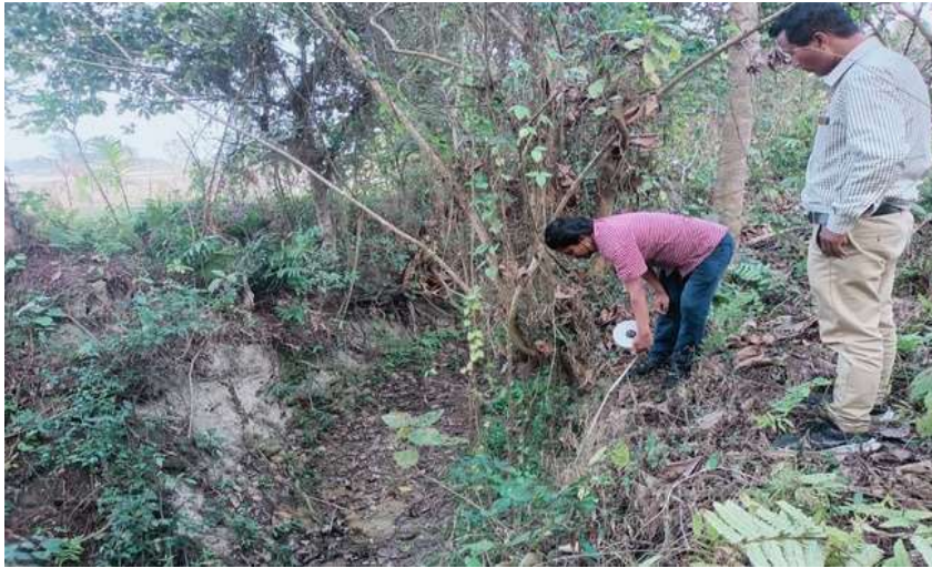
Gully Control Project at Dhupguri MWS-3
